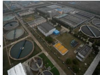
Nanjing wastewater treatment facility, China
