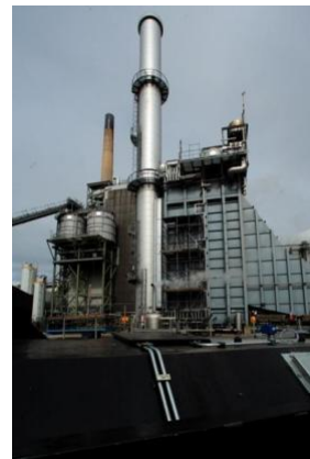
Sembcorp Biomass Power Station, UK
