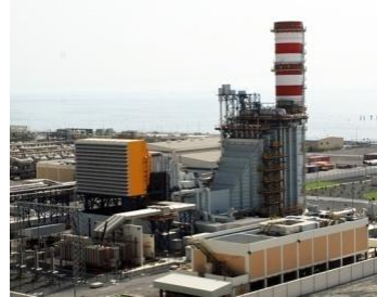
Fujairah Independent Water and Power Plant, UAE
