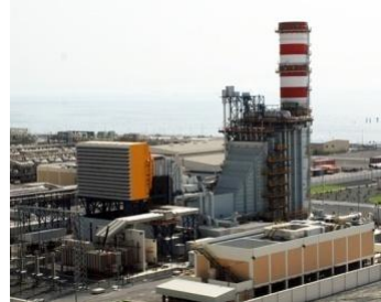
Fujairah Independent Water and Power Plant, UAE
