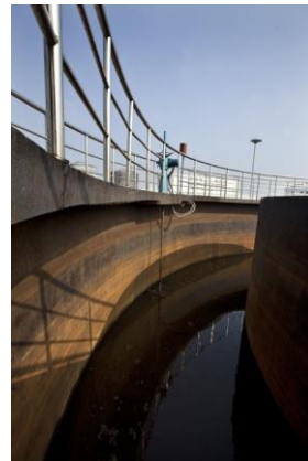
Zhangjiagang wastewater treatment facility, China
