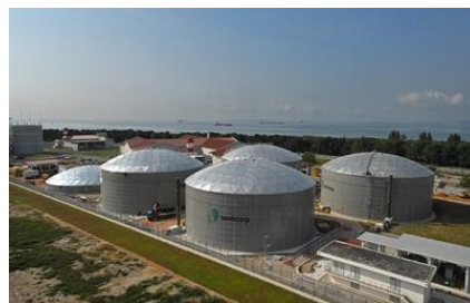
Sembcorp NEWater Plant, Singapore
