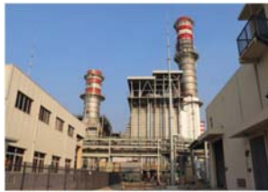
Sirajganj Unit 4 power plant, Bangladesh
