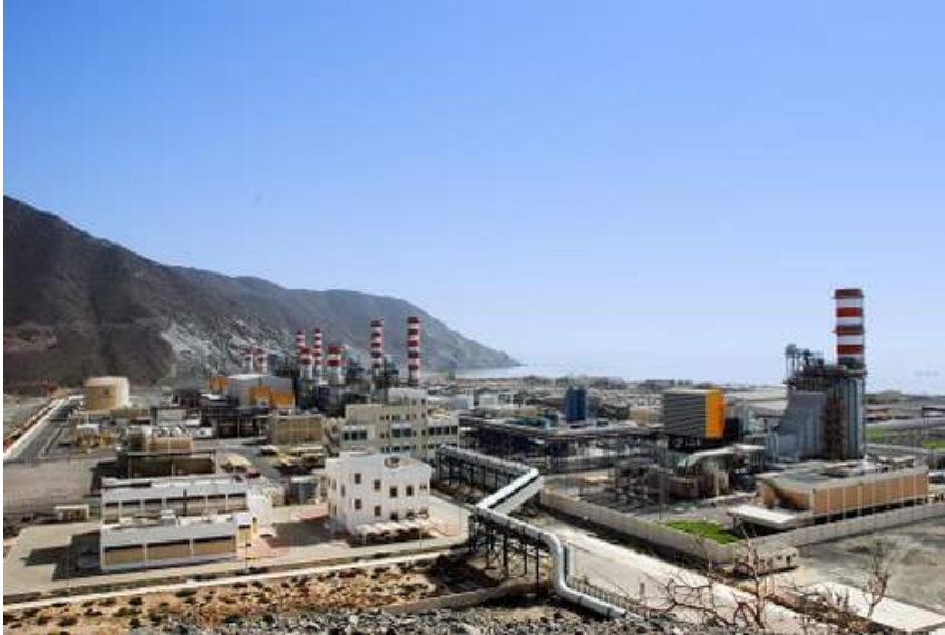
Pictured above: Sembcorp has expanded power capacity at its Fujairah combined power-and-desalination plant by over 40%.
